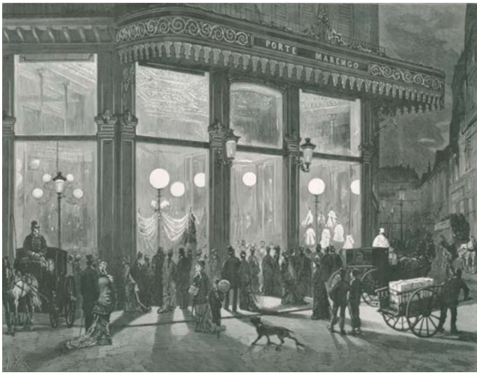
The Porte Marengo display window
